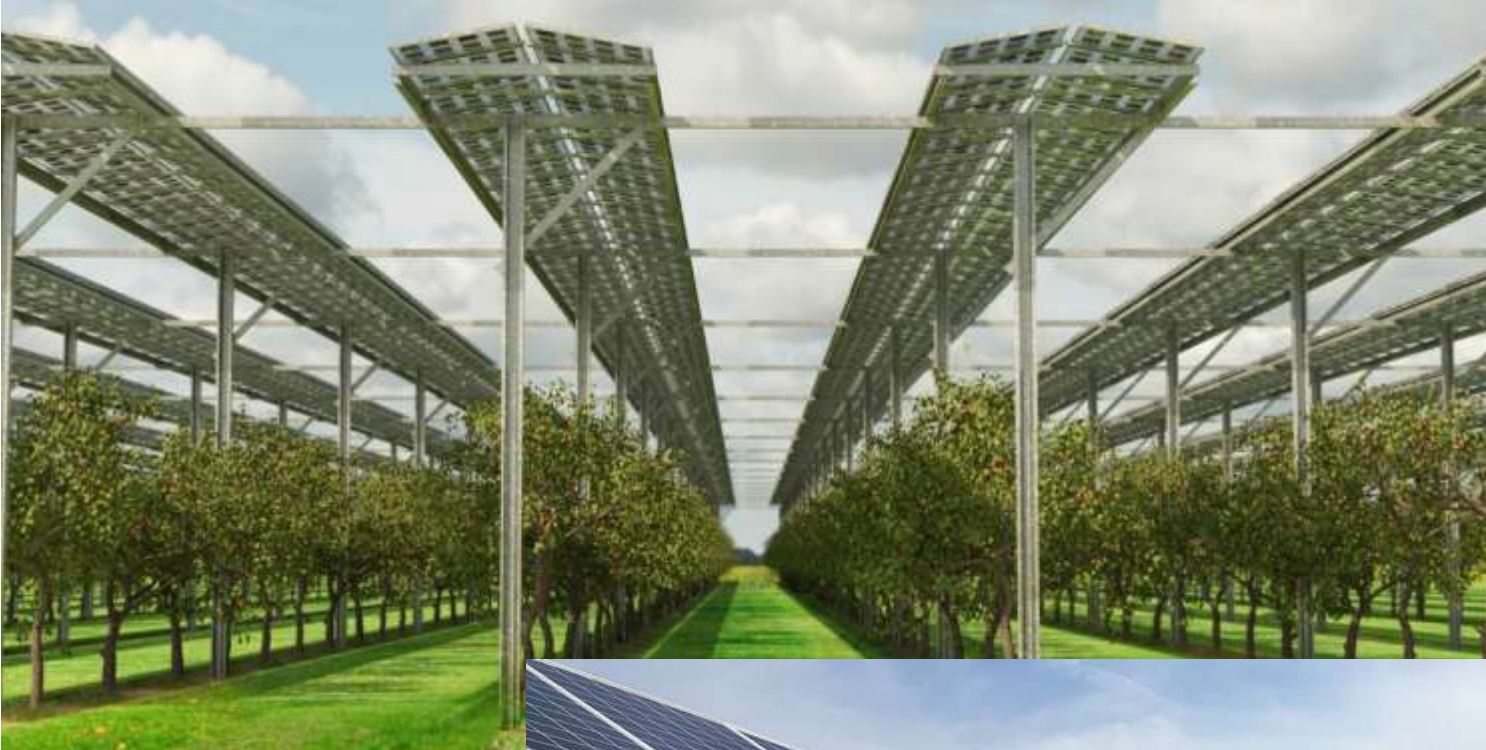
FlexAgri Fruit Solar Structure Design for Agrivoltaics and Fruit Trees (Voestalpine SadeF)
