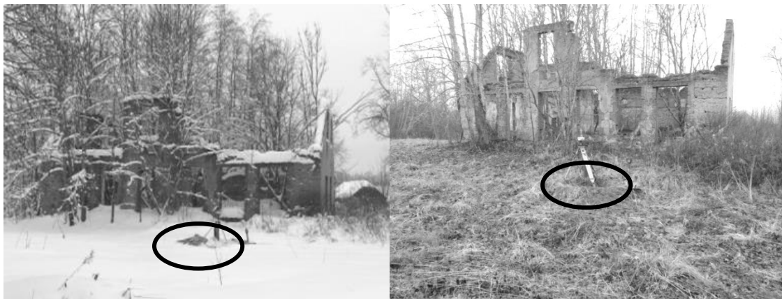
Fig. 2. Class I leveling network point No. 1484 in 2012 (left) and in 2013 (right).
